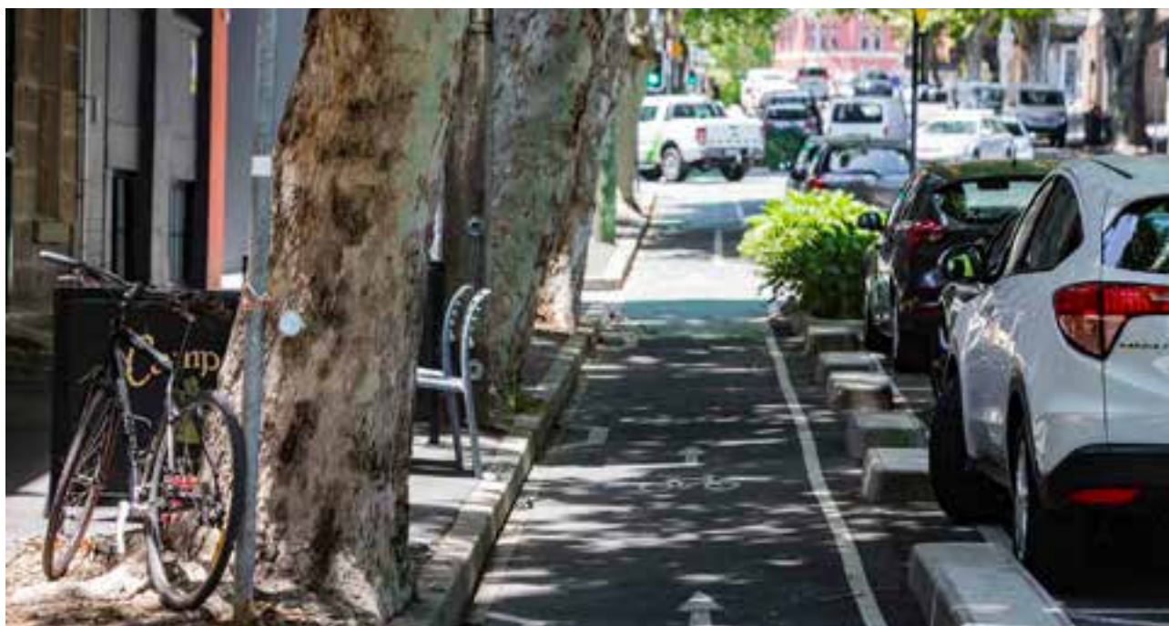
Figure 3.8 Bicycle path (one-way), Campbell Street, Surry Hills
