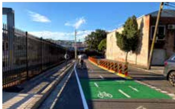
Figure 6.6 Pop-up facilities should be provided along routes that are designated as part of any future permanent network, including connectivity with other modes of transport to enable ease of interchange.
