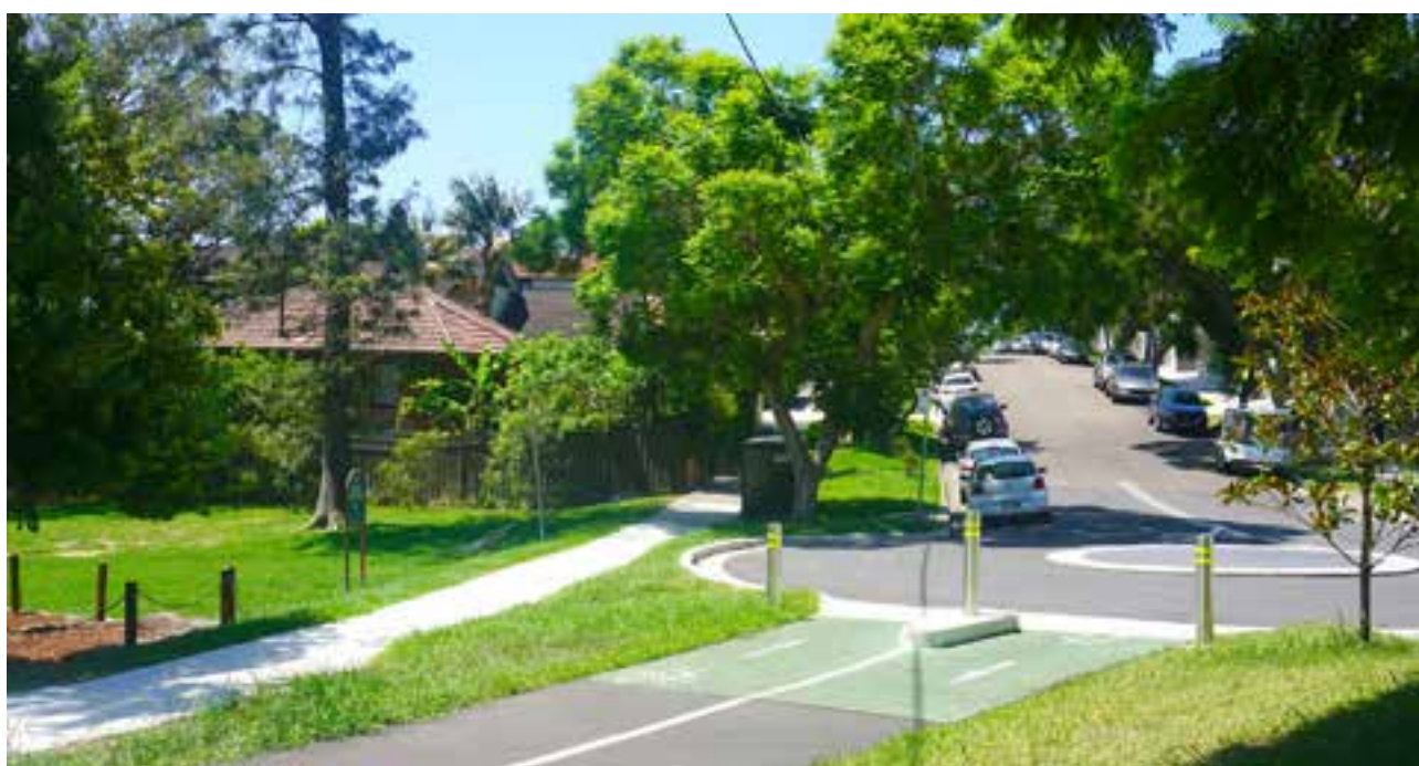
Figure 3.47 Modal filter, Ellalong Road, Cremorne
