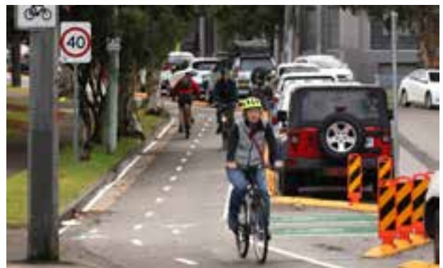
Figure 6.4 Pop-up cycleway facilities, like this one on Henderson Road, can be constructed quickly and with limited or no permanent changes to the road surface (Credit: Transport for NSW)
