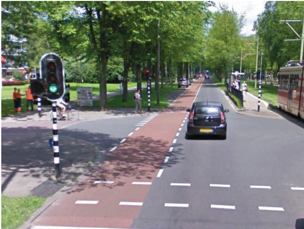
Figure 51: Dutch on-road bicycle lane painted red through signalised intersection, Delft, Netherlands
