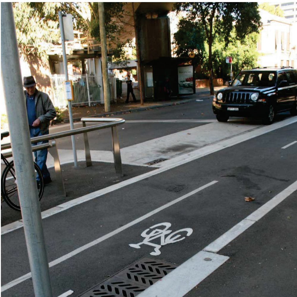
Figure 19: Dual kerb two-way cycle track with drainage pits at both kerbs, Bourke St, Sydney
