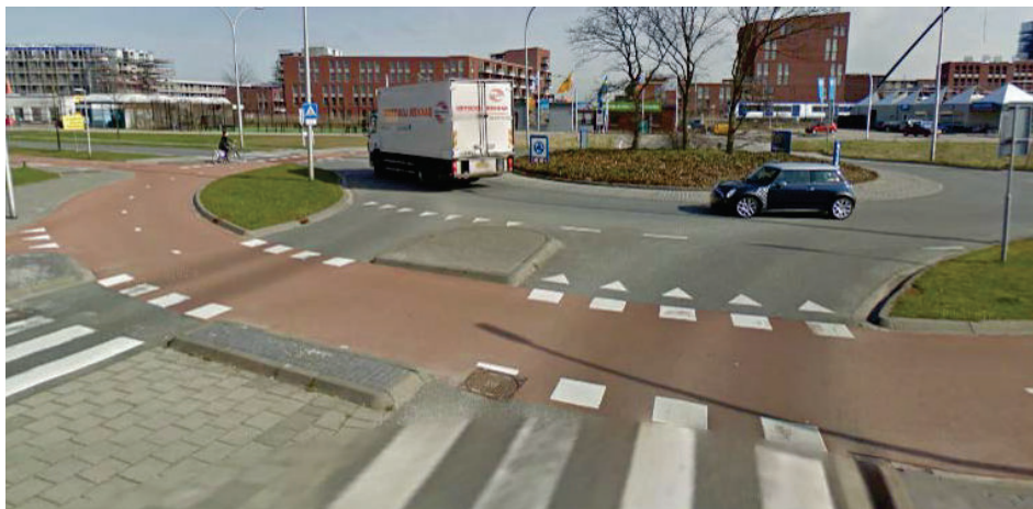
Figure 43: Pedestrian and bicycle priority crossings at a single lane roundabout, Pijnacker, Netherlands
