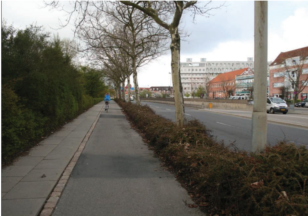
Figure 10: One-way cycle track on arterial road, Odense, Denmark
