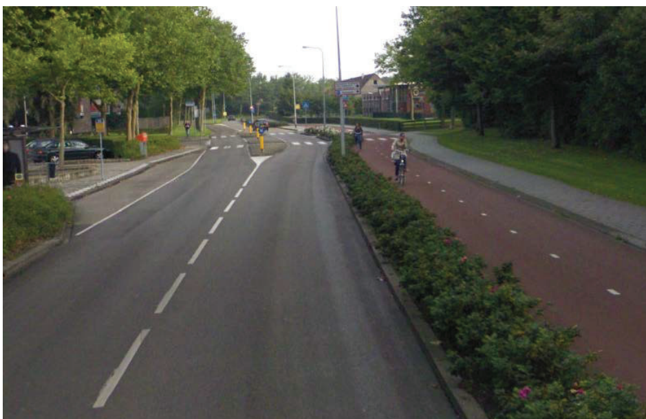
Figure 15: Two-way cycle track, Groningen, Netherlands
