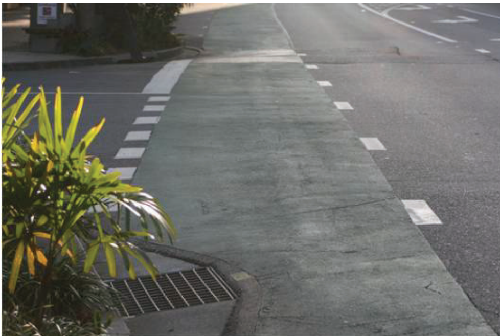
Figure 28: Bicycle lane with priority at side road, Brisbane
