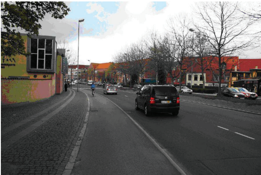
Figure 3: One-way cycle track on arterial road, Odense, Denmark
