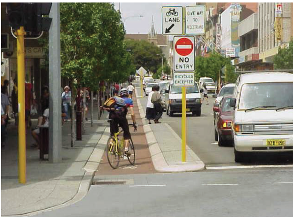
Figure 17: Contra-flow one-way cycle track, Perth
