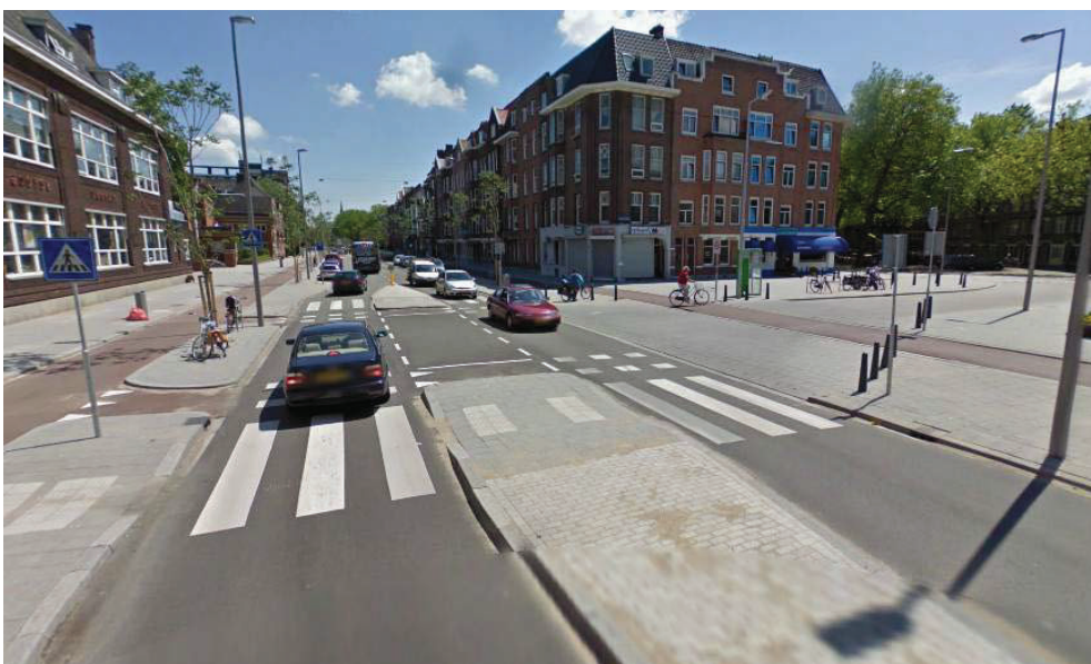
Figure 67: One-way cycle track on collector road with pedestrian crossings and refuges, Rotterdam Holland in street view (refer to Figure 66)
