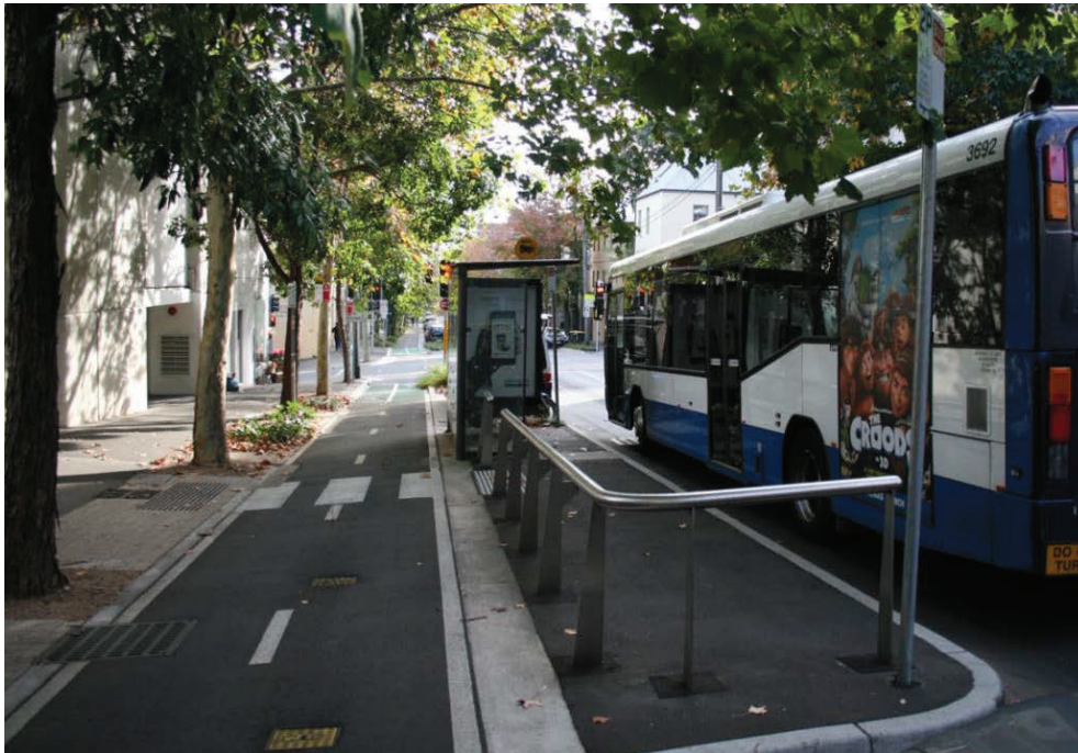
Figure 65: One-way cycle track at bus stop, Copenhagen
