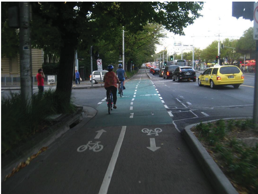
Figure 27: Two-way cycle track with priority crossings, not raised, Melbourne. Note the turning restriction during certain times for motor vehicles
