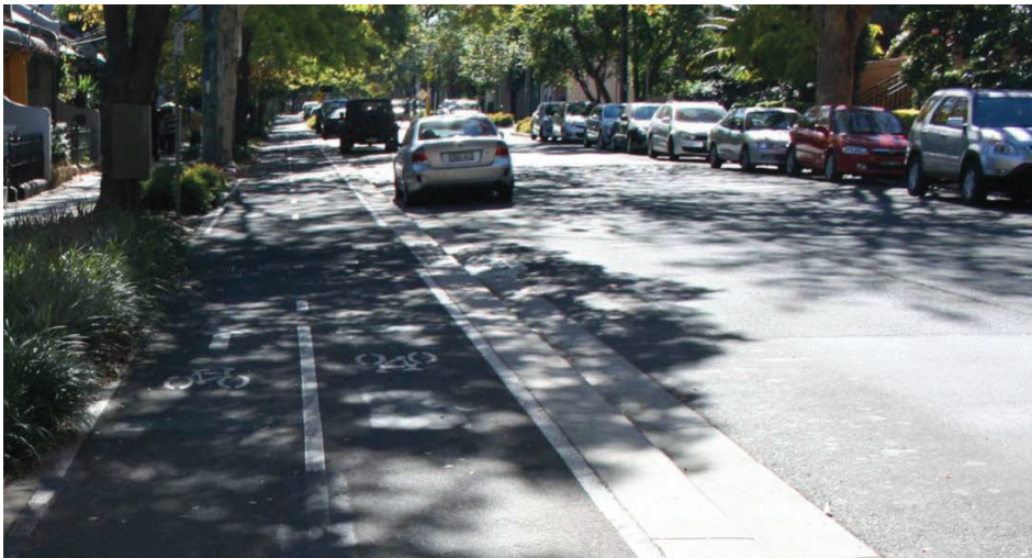
Figure 14: Two-way cycle track, Bourke St, Sydney
