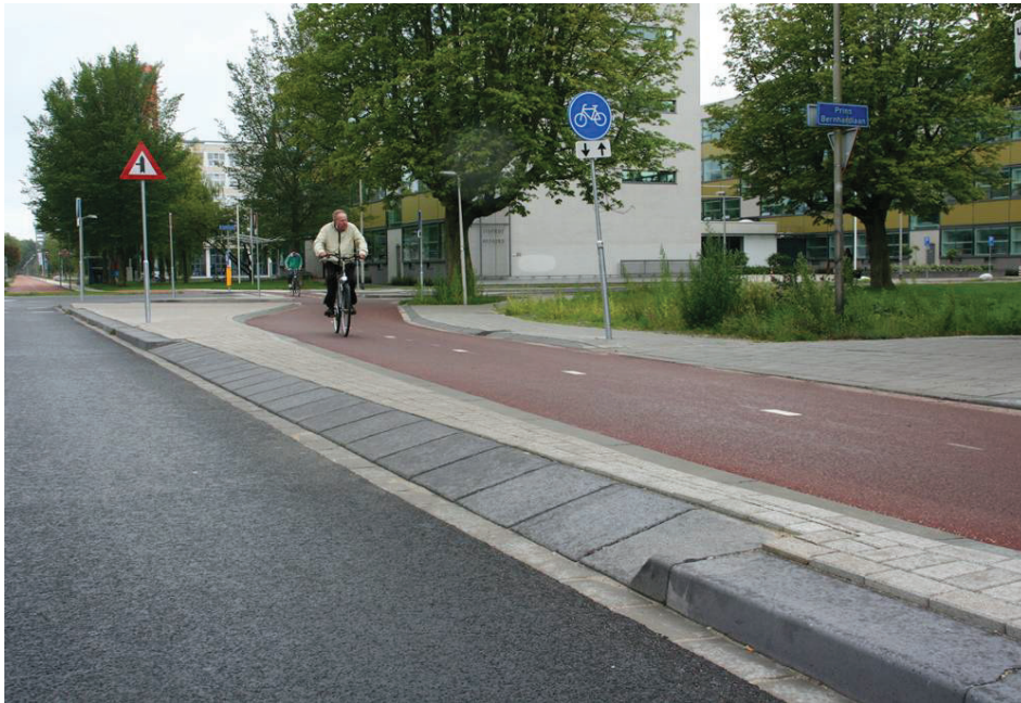
Figure 31: Example of Dutch ‘exit construction’ (1 in 4 gradient mountable kerb) at a two-way cycle track raised priority crossing at side road
