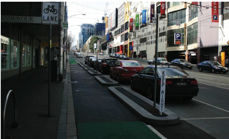
Figure 12: One-way cycle track with parking, with at-grade footpath at side road, Latrobe St, Melbourne
