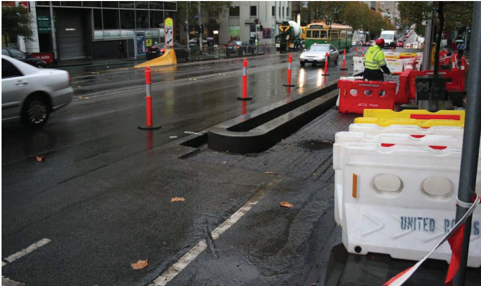
Figure 13: One-way cycle track under construction, Latrobe St, Melbourne
