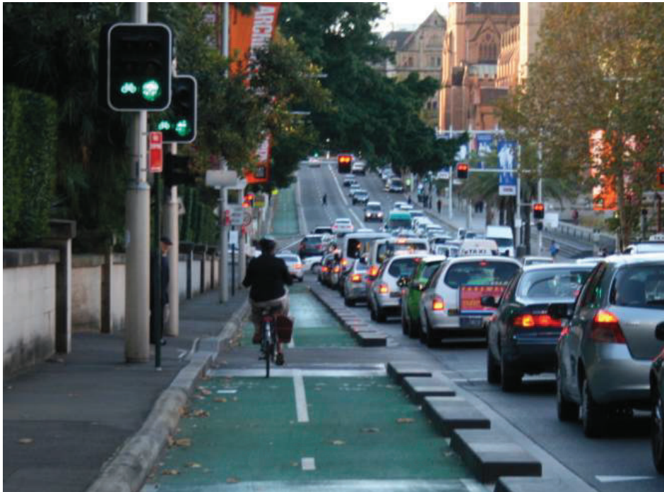
Figure 16: 2.4 m wide two-way cycle track with 0.4 m separator and no parking, College Rd, Sydney
