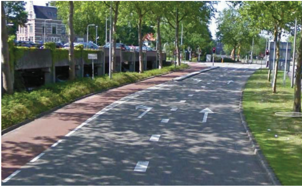
Figure 52: Dutch on-road bicycle lane transitioning to cycle track at signalised intersection, Delft, Netherlands
