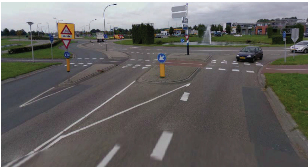
Figure 47: Urban multiple lane roundabout with priority crossings on one leg, Rotterdam, Netherlands
