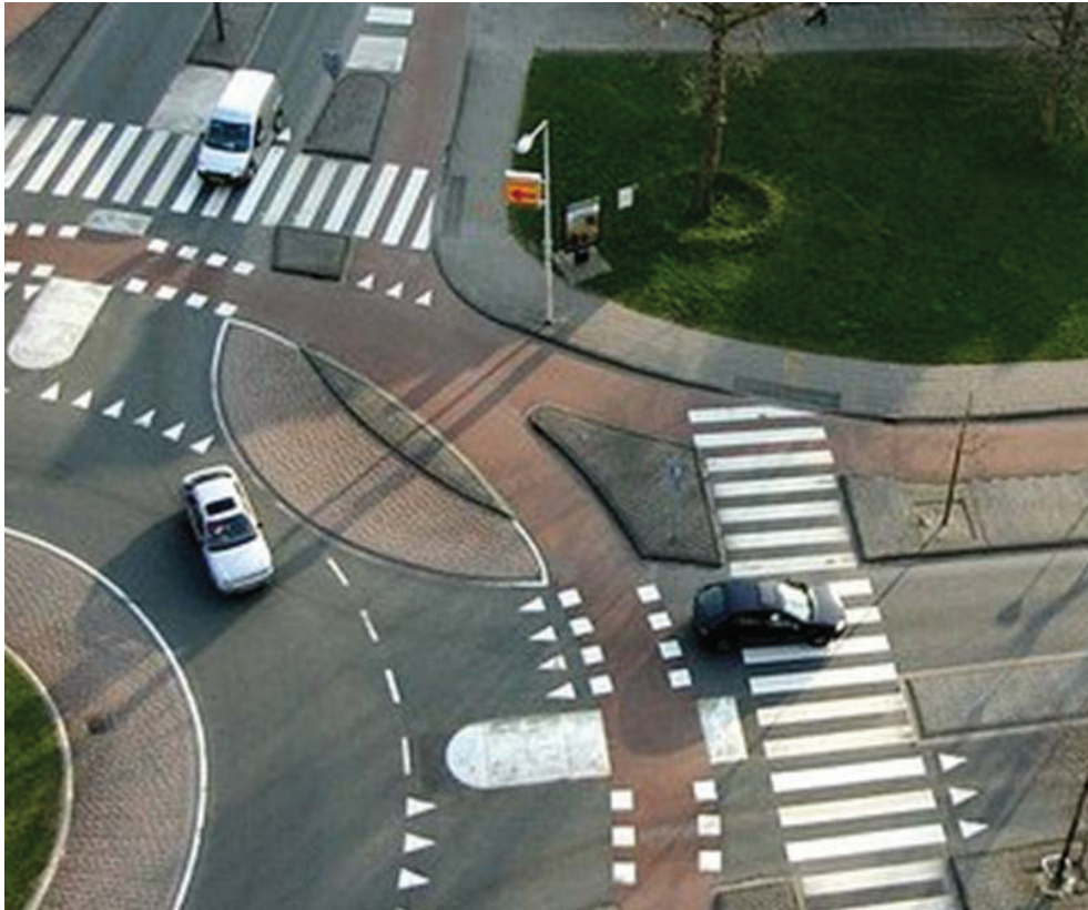
Figure 40: Dutch single lane roundabout, separated cycle track, priority crossings, not raised. See appendix for detailed design. Includes 'sharks teeth' give-way line marking which is currently not approved for use in Queensland
