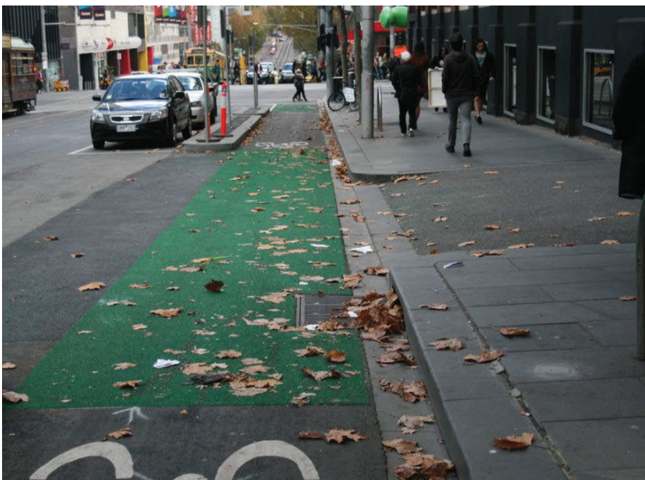
Figure 12: One-way cycle track with parking, with at-grade footpath at side road, Latrobe St, Melbourne
