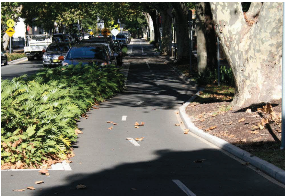
Figure 63: Two-way cycle track diverted around existing street tree, Bourke St, Sydney
