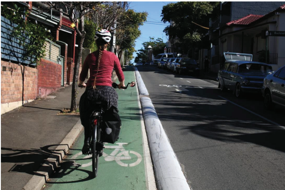
Figure 9: Contra-flow bicycle lane with semi-mountable kerb separation, George St, Sydney
