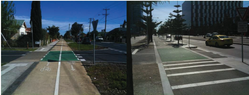
Figure 33: Two-way cycle tracks with raised priority crossings at side roads, Melbourne
