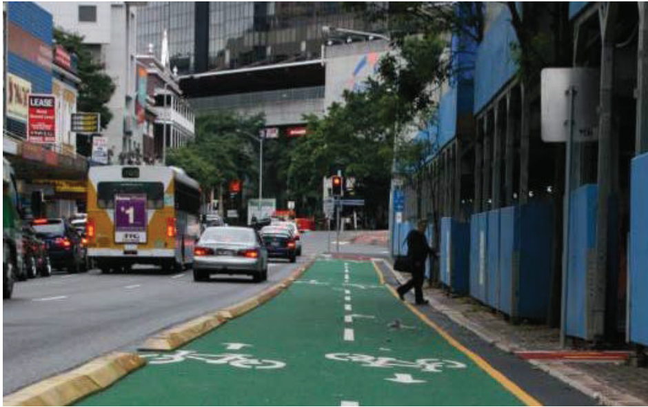
Figure 23: One-way cycle track on 2-way multilane road, median separated profile, Latrobe St, Melbourne. This example shows 1.1 m median with parking and further down a 0.3 m median where there is no parking
