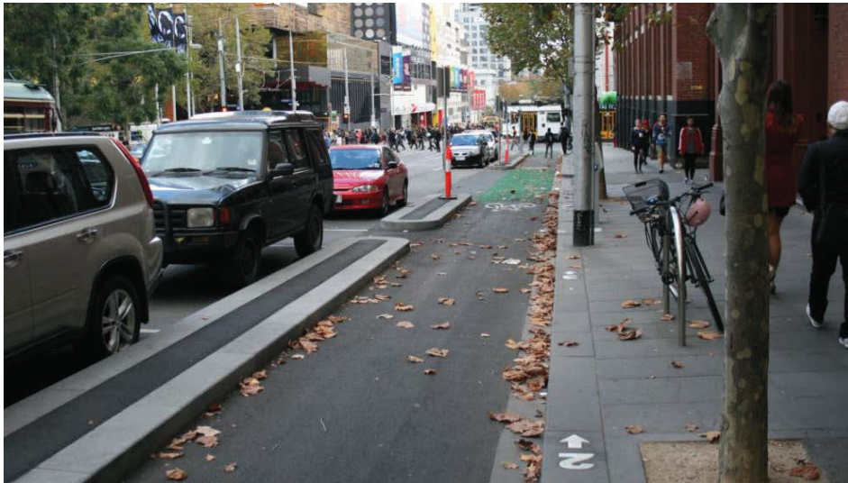
Figure 21: Two-way cycle track, median separated profile. Sydney
