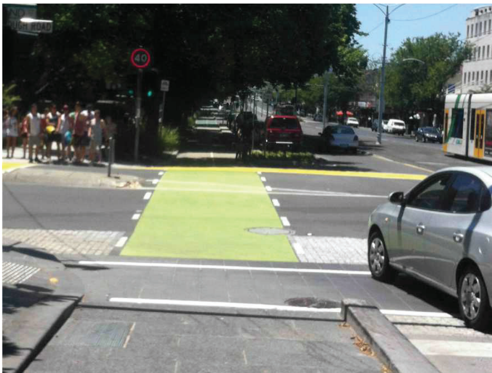
Figure 50: Two way cycle track signalised intersection. Fitzroy Street, St Kilda, Victoria
