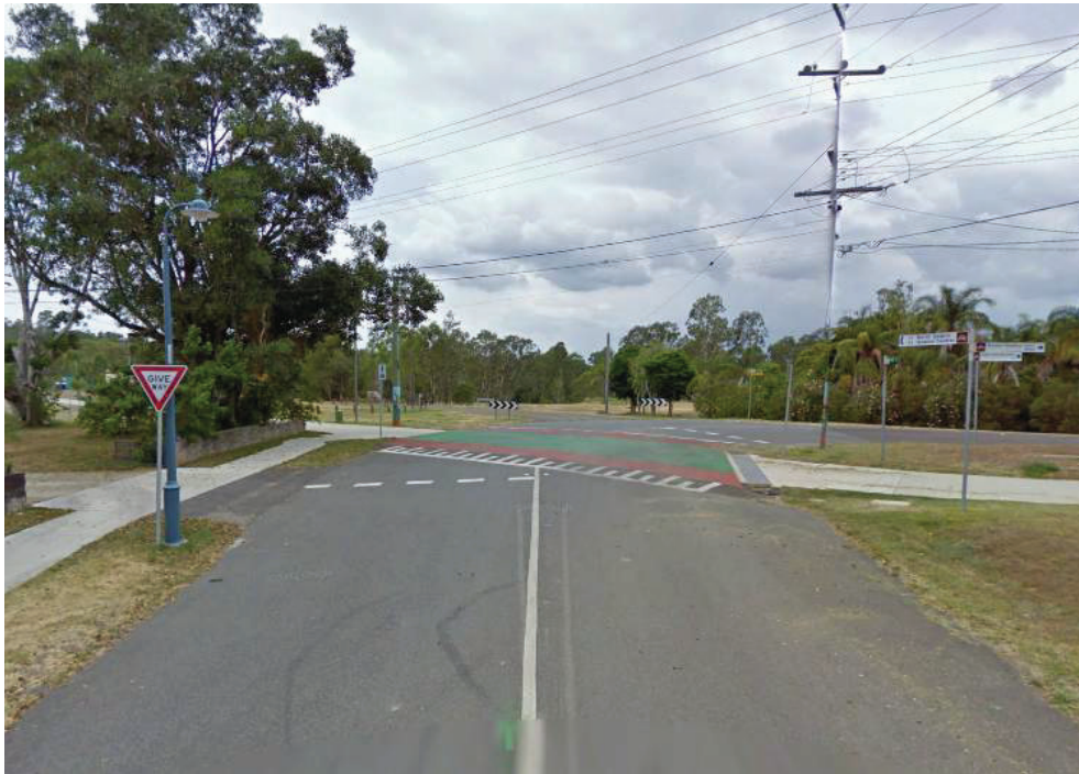
Figure 37: Mid-block shared path raised priority crossing, Ipswich, Queensland
