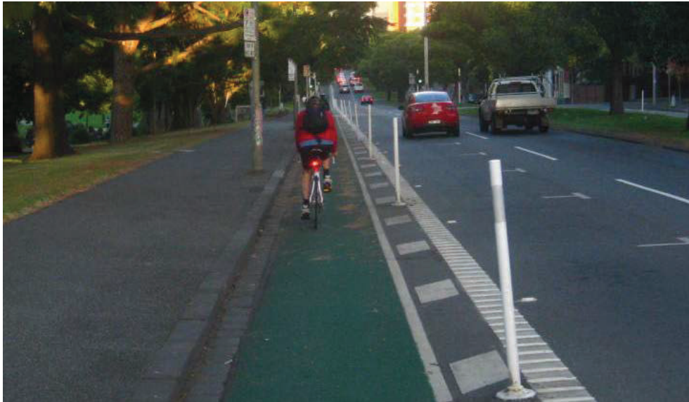
Figure 7: Buffered bicycle lane with off-peak parking, Albert St, Melbourne
