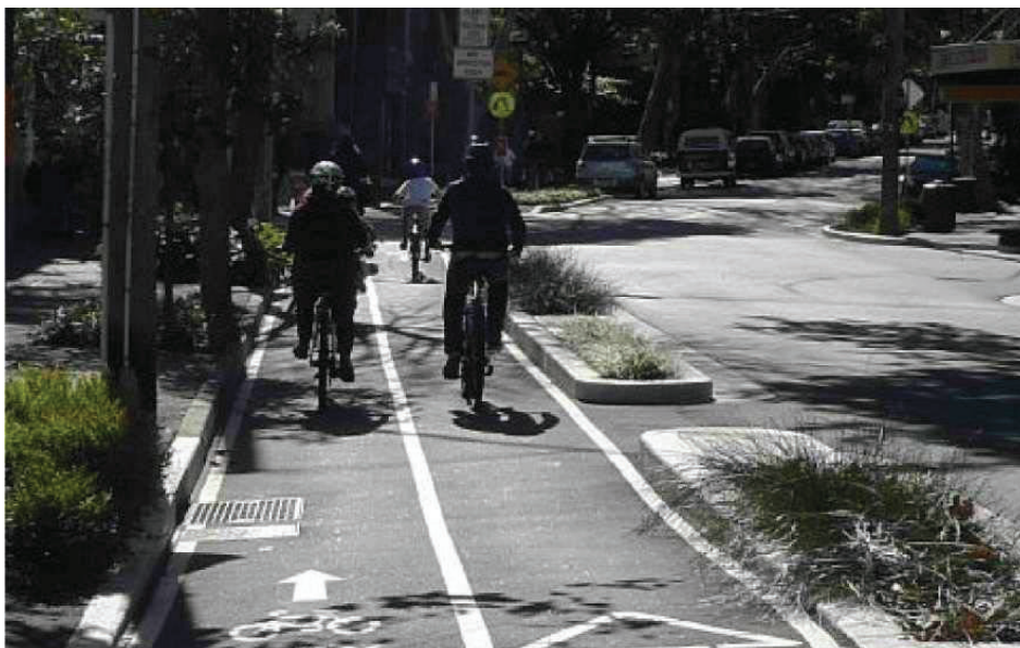
Figure 21: Two-way cycle track, median separated profile. Sydney
