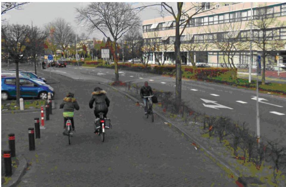
Figure 4: Service road designed for low speed (30 km/h), Voorburg, Netherlands
