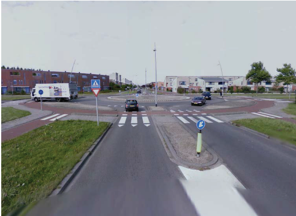
Figure 41: Pedestrian and bicycle priority crossings at a single lane roundabout, Groningen, Netherlands
