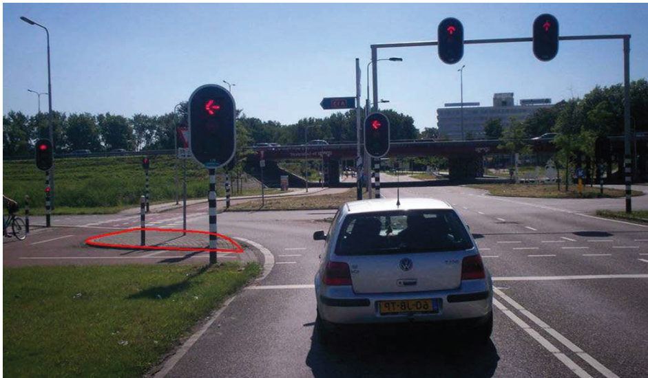
Figure 58: Arterial road (limited access) crossing a two-way cycle track, with corner island circled in red. This intersection is time separated by signals triggered in advance by bicycle riders to reduce the chance of stop
