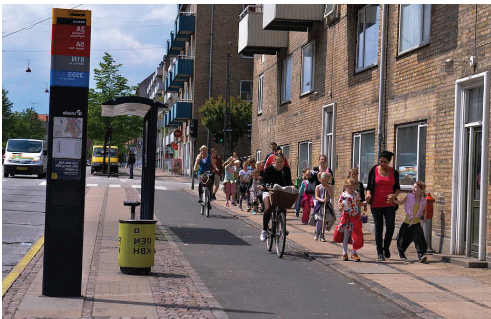
Figure 65: One-way cycle track at bus stop, Copenhagen
