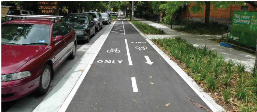
Figure 25: Two-way cycle track, one-step profile. Bourke St, Sydney
