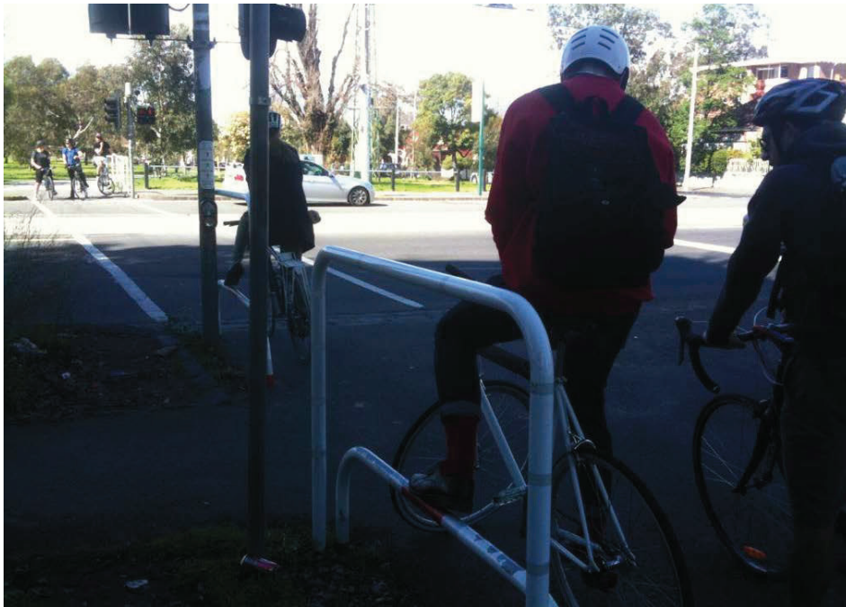
Figure 60: Holding rails and foot rails for comfortable waiting at signalised crossing, Melbourne
