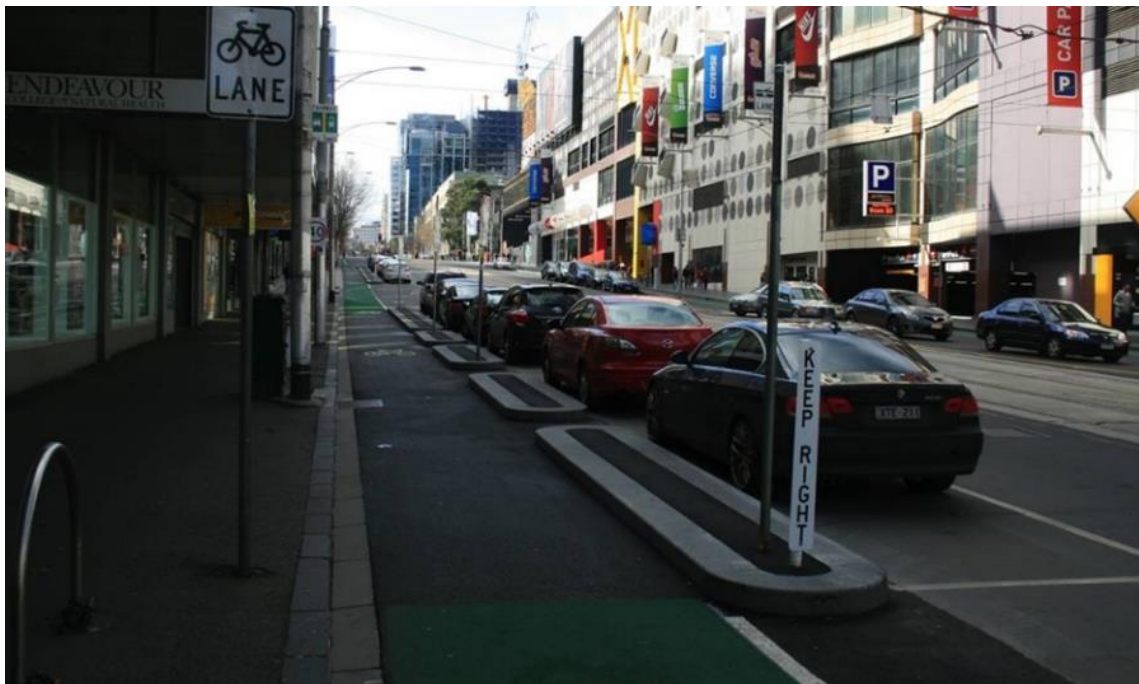
Figure 3.2.1(B) – One-way cycle track with parking, with at-grade footpath at side road, Latrobe Street, Melbourne
