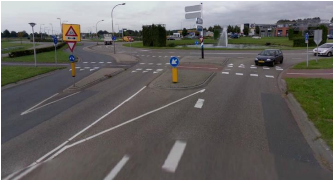
Figure 4.4.3(A) – Large multiple-lane roundabout with priority crossings for two-way cycle track crossing one lane at a time, on one leg only, Rotterdam, Netherlands (LTS2)
