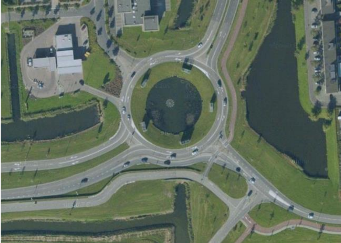
Figure 4.4.3(B) – Urban multiple lane roundabout, Rotterdam, Netherlands (LTS2)
