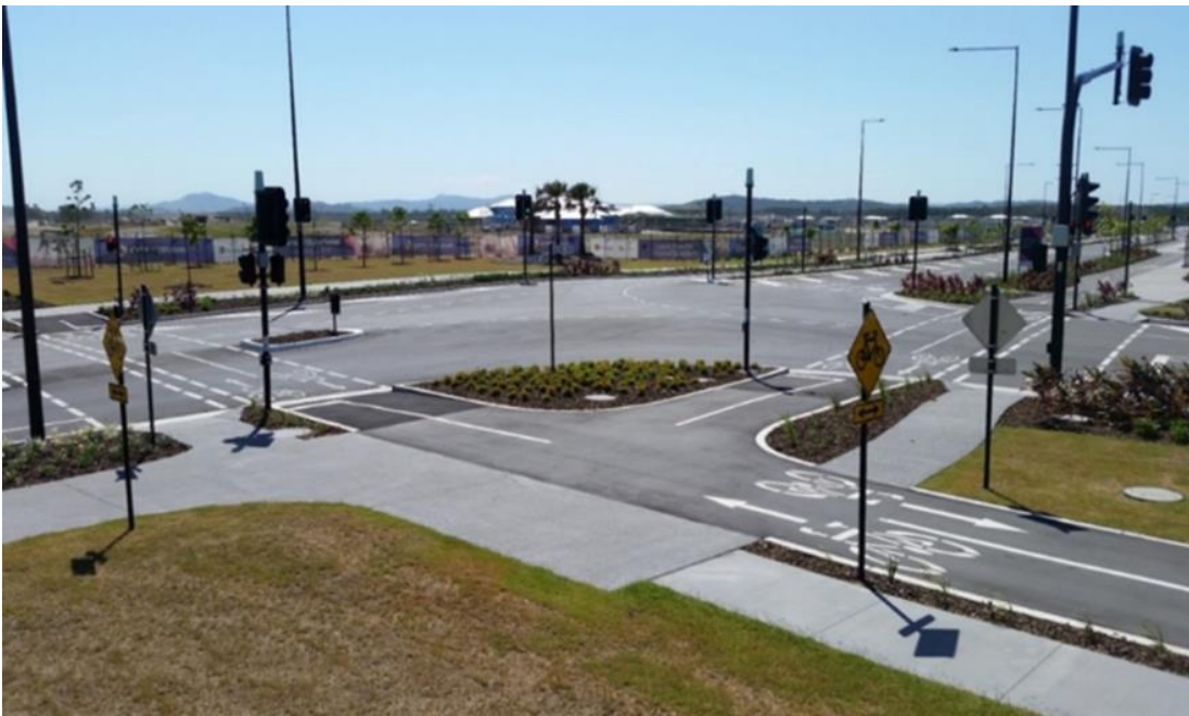
Figure 4.5(A) – Protected signalised intersection with two-way cycle tracks. Aura, Caloundra
