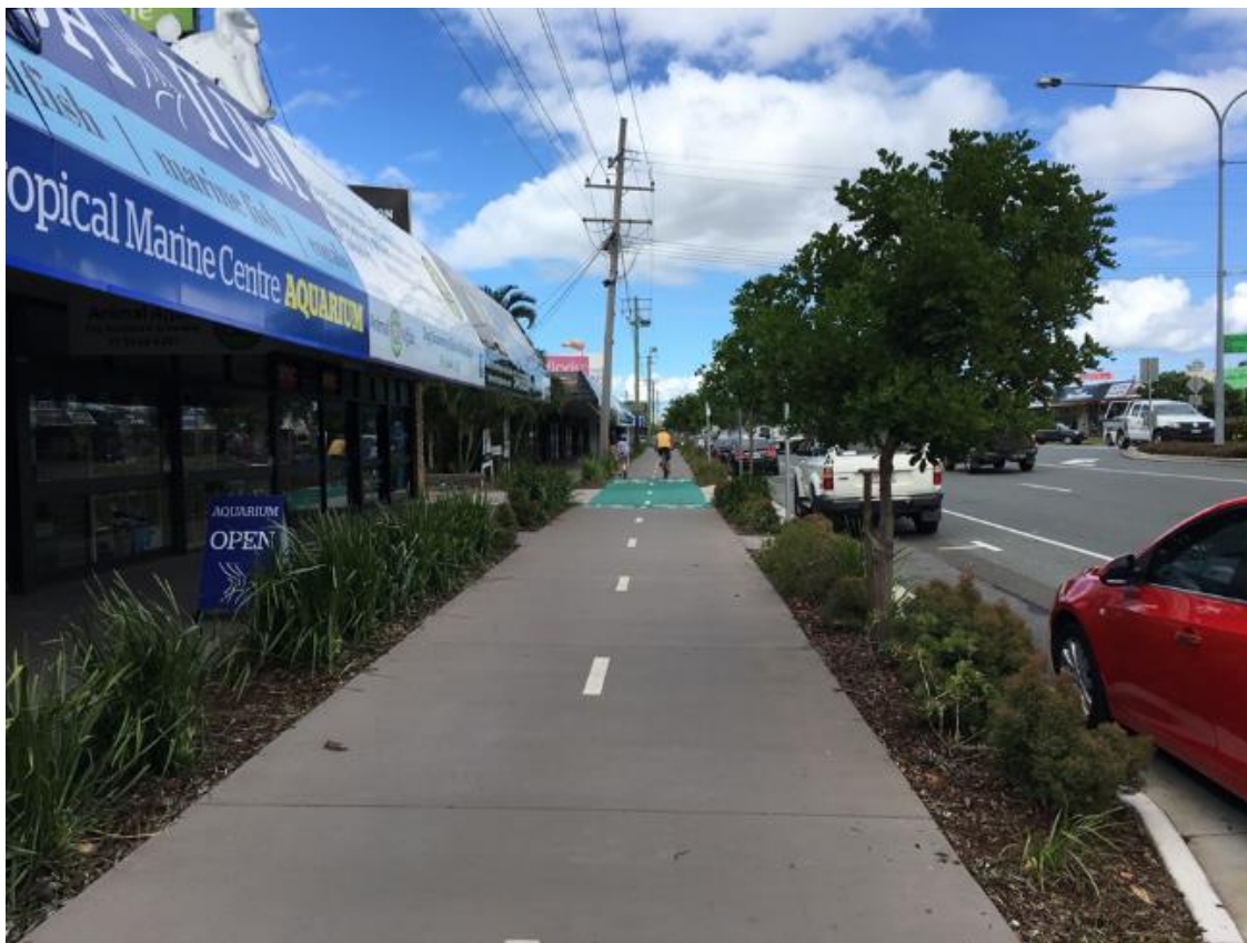
Figure 3.3.4(A) – Planting separation between cycle track and footpath, Brisbane Road, Mooloolaba
