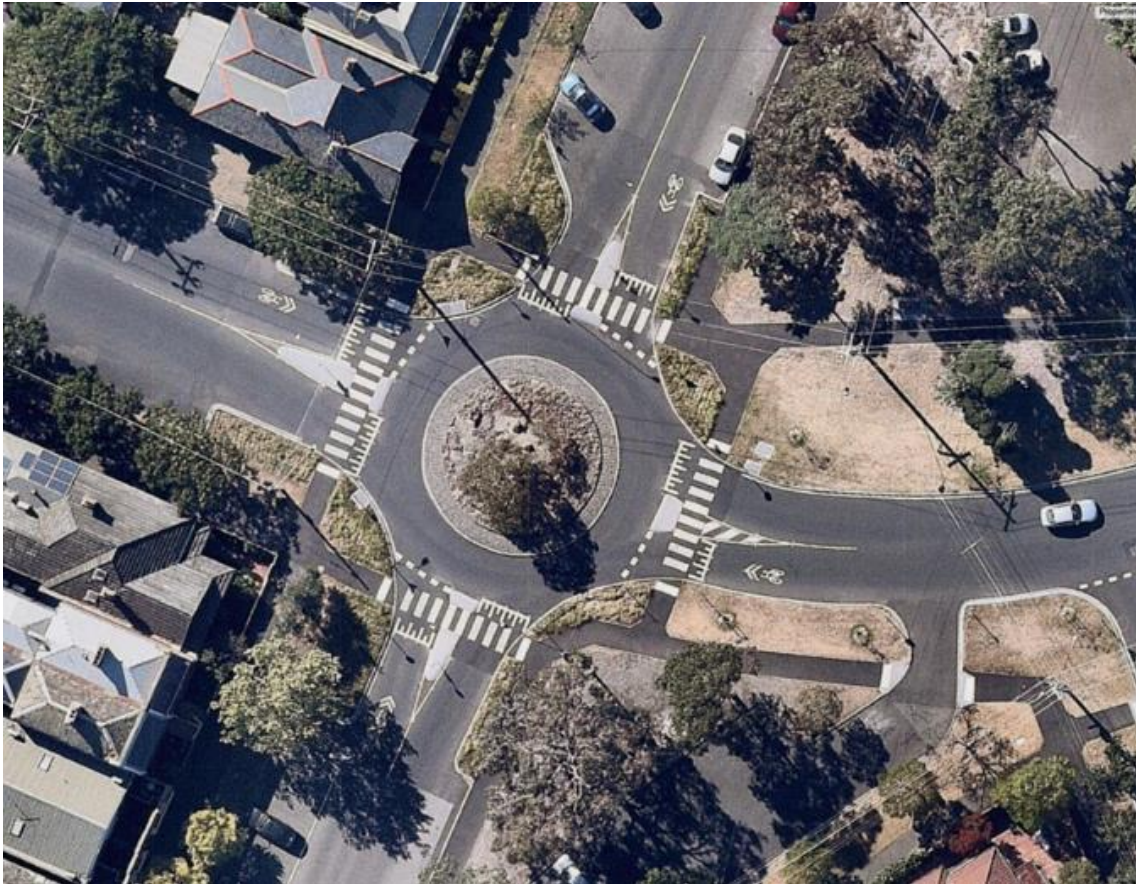
Figure 4.4.1(A) – Mixed single lane roundabout with zebra crossings on all approaches and mountable apron on centre island, Nelson Road, South Melbourne (LTS2)
