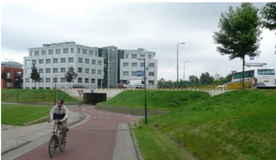
Figure 4.4.2(C) – Grade-separated roundabout, Houten, Netherlands (LTS1)
