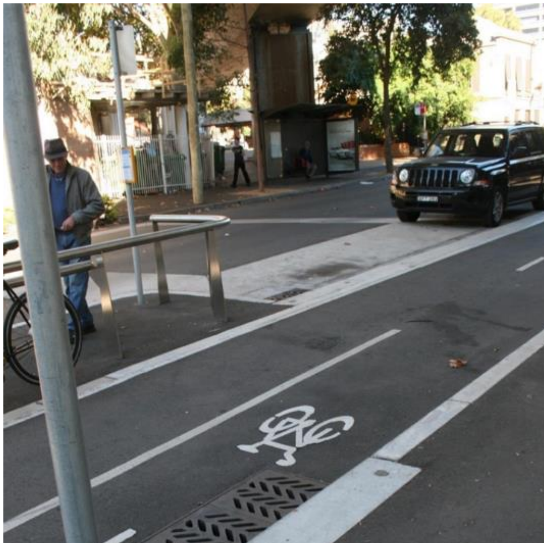
Figure 3.2.6.1(B) – Dual kerb two-way cycle track with drainage pits at both kerbs, Bourke Street, Sydney
