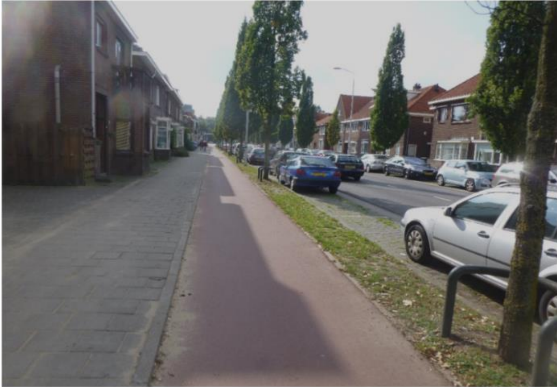
Figure 3.2.1.1(C) – One-way cycle track and parking, Nijmegen, The Netherlands (5.0 m total width)
