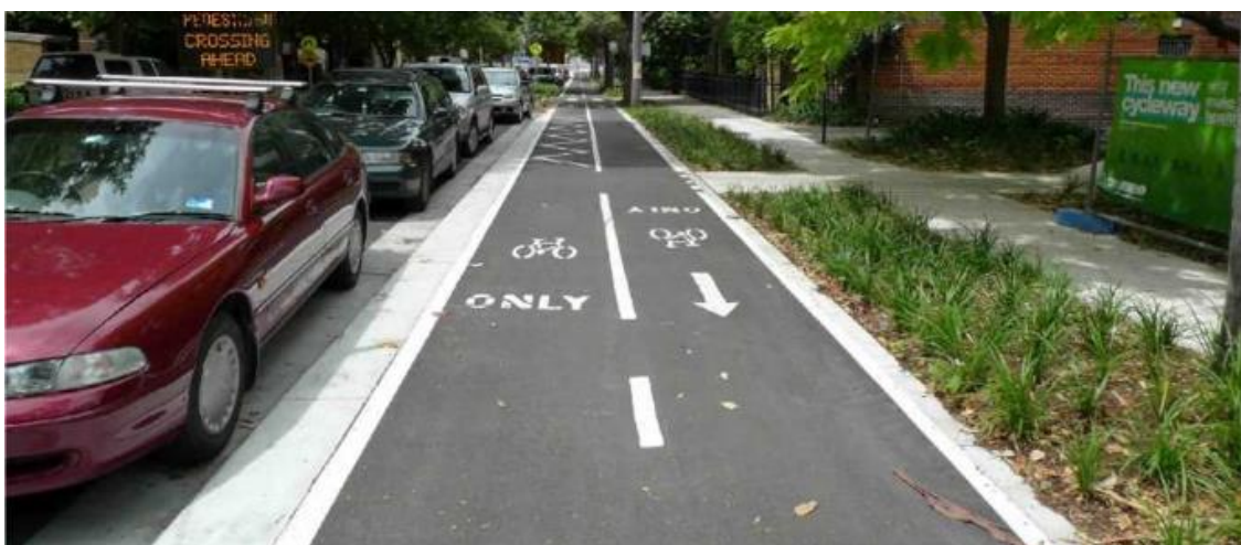
Figure 3.2.6.3(A) – Two-way cycle track, one-step profile – planting separation and pavement contrast. Bourke Street, Sydney
