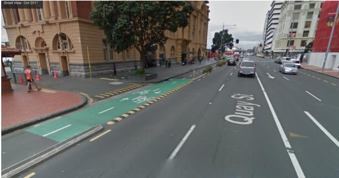
Figure 4.3.1(D) – Low cost retrofit treatment side street Quay Street, Auckland (LTS2)
