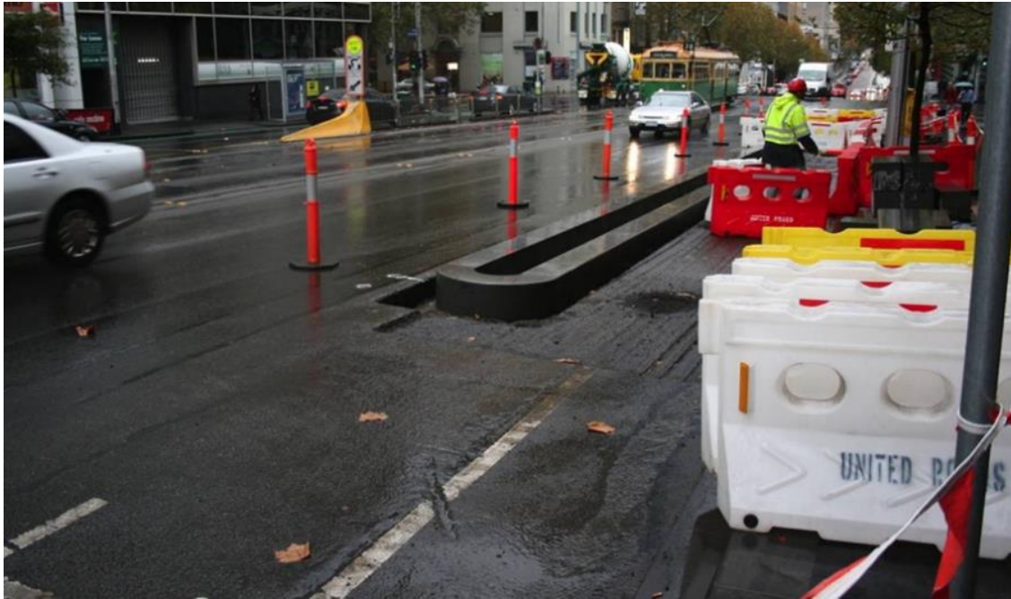
Figure 3.2.1(C) – One-way cycle track under construction, Latrobe Street, Melbourne
