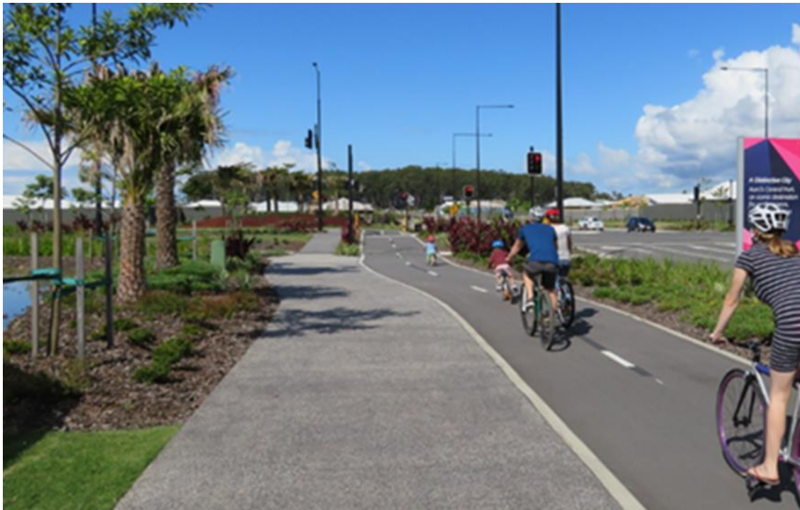
Figure 3.3.4(B) – Pavement difference between cycle track and footpath, Aura, Caloundra
