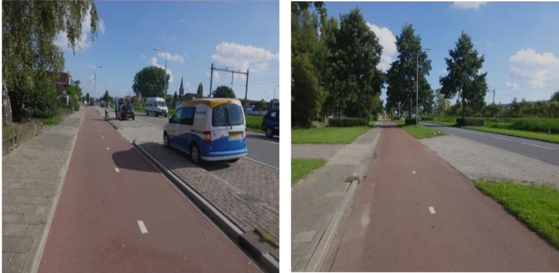
Figure 4.7.3 – Two-way cycle track crossing residential driveway, Rotterdam
