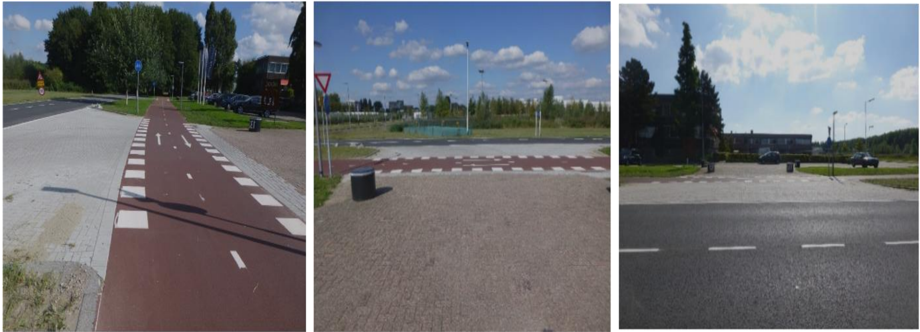
Figure 4.7.2(A) – Three angles of a two-way cycle track crossing industrial area driveway, Rotterdam
