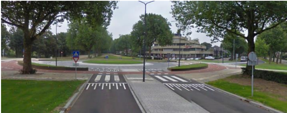
Figure 4.4(A) – Single-lane roundabout, motor vehicle entry and exit angle 90°, two-way cycle track with raised priority crossings and zebra crossings for pedestrian priority, Den Bosch, The Netherlands (LTS1)
