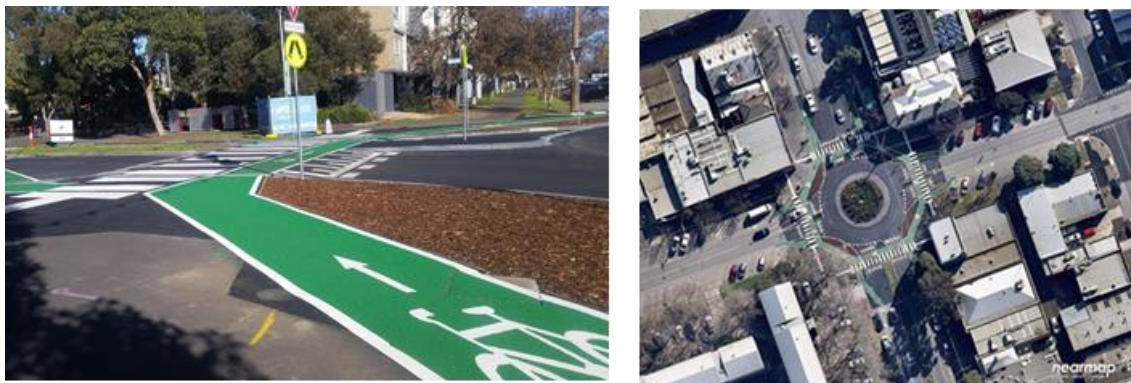
Figure 4.4.1(C) – Retrofitted protected roundabout intersection with raised zebra and cycle track crossings, Moray Street / Dorcas Street, South Melbourne (LTS1)
