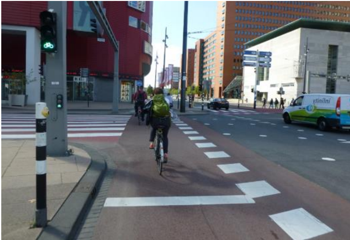
Figure 4.5.2(G) – Push button conveniently located 200 mm from cycle track at signalised intersection with advanced stop line, Rotterdam
