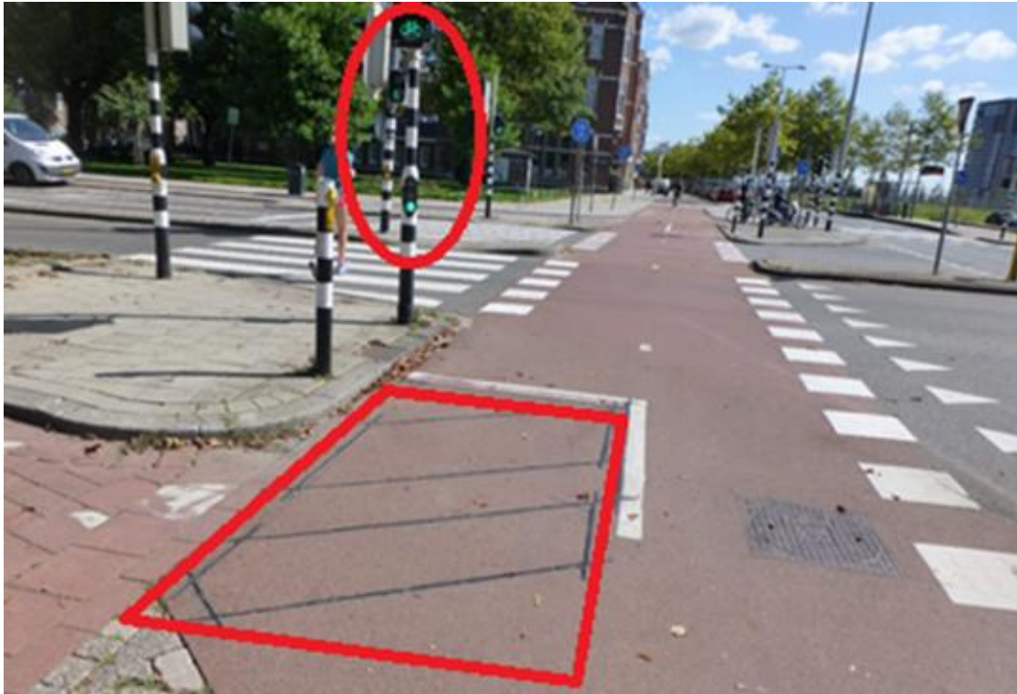
Figure 4.5.2(F) – Three aspect lanterns and detection loops locations, Rotterdam, The Netherlands
