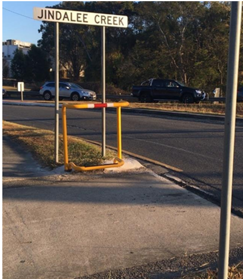
Figure 4.5.1(H) – Holding rails and foot rails for comfortable waiting at signalised crossing, Jindalee
